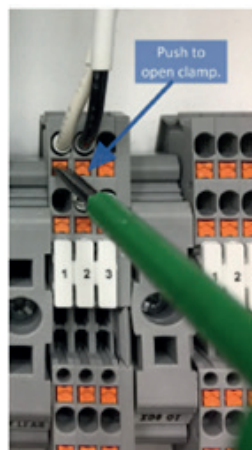
Figure 37. Opening terminal block clamp
